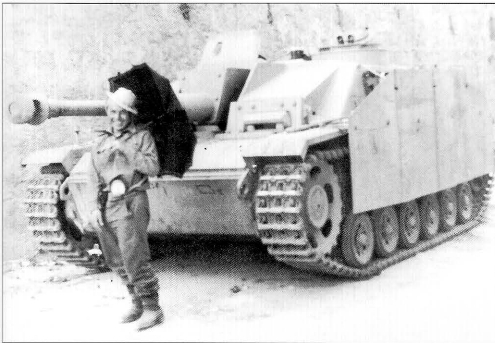
One of the crewmen of this StuG.III Ausf.G from 16.Panzer-Division, strikes a jaunty pose for the camera. This is one of the StuG.III Ausf.G manufactured from PzKpfw.III Ausf.M chassis by M.A.N. between January and March 1943 and features the welded 30mm additional armor plates on the front of the hull and one piece hatches on the glacis. Note the longer deflector in front of the driver's visor. The tactical sign for a Panzer Kompanie is painted on the front plate followed by a '3', probably in black.
