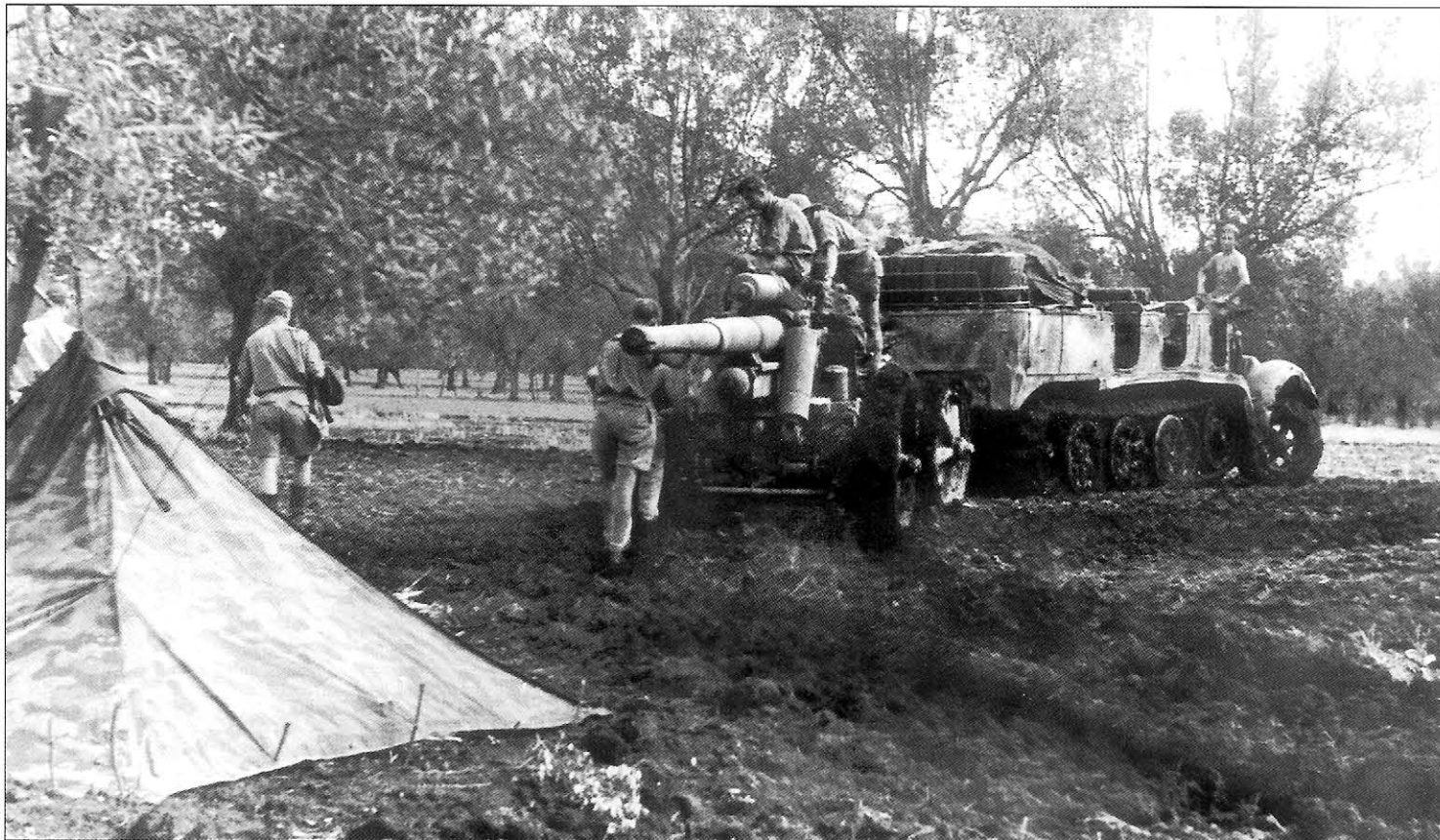
A 15cm sFH18 artillery gun towed by an Sd.Kfz.7 half-track, is maneuvered around a grove of trees being used as a camp by a heavy towed artillery unit. The Zeltbahn camouflage shelter quarter was designed to be joined together with others to form a small tent. The Sd.Kfz.7 is finished in overall dark yellow with a camouflage paint scheme of green patches.
