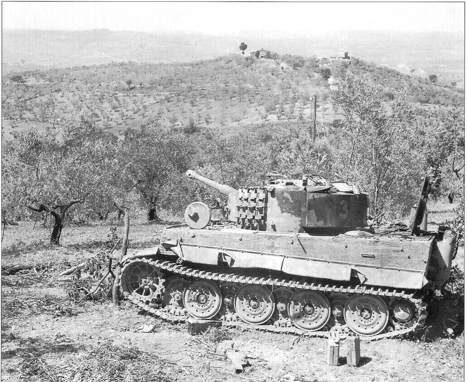
A late Tiger I Ausf.E from 3./s.Pz.Abt.508 sits abandoned in a grove of olive trees, the rear of its turret blackened by an engine fire. The white outline tactical number '3' is still plainly visible on the side of the turret and rear of the stowage bin. The 3.Kompanie was equipped with Borgward BIV radio controlled demolition vehicles and so these Tigers had an additional radio antenna mount added to the right side of the turret.
