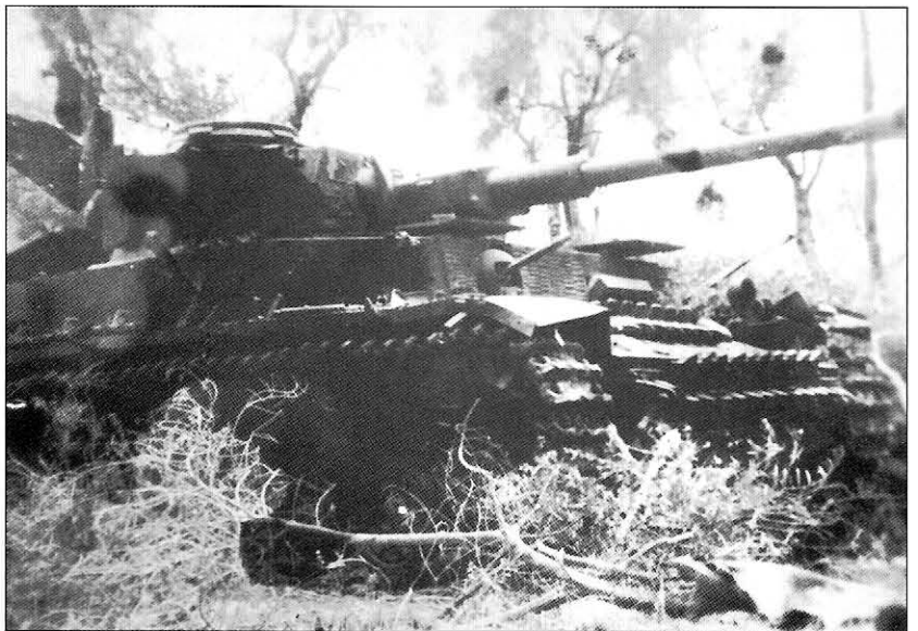
This Pz.Kpfw.IV Ausf.H was knocked out in the Cassino area in early 1944. By this time, most new armored vehicles were being delivered with Zimmerit anti-magnetic mine coating which is visible here on the superstructure front plate.
