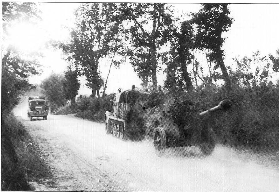
The Sd.Kfz.11 light 3-ton half-track prime mover was employed for towing a variety of light howitzers, anti-tank guns and the Nebelwerfer rocket launcher. Here, an Sd.Kfz.11 is towing a 7.5cm PaK40 anti-tank gun along a dusty country road. The gun crew has added some cut foliage to the gunshield for camouflage.
