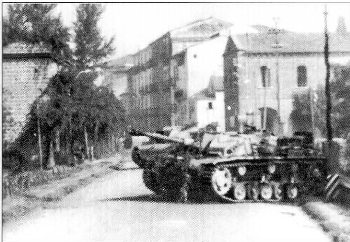
Two StuG.III Ausf.G from an unidentified unit parked along an Italian street. The nearest vehicle is fitted with the smoke grenade launchers installed on vehicles manufactured from February to May 1943.
