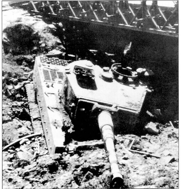
This Tiger I Ausf.E from s.Pz.Abt.508 bogged down and had to be abandoned while trying to cross a soft streambed. In order to avoid the same fate, the Allies have erected a Bailey Bridge across the obstacle.
