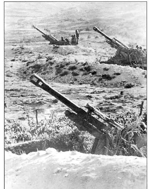
Stablemate of the Hummel, the Wespe mounted the 10.5cm IFH18M howitzer on the obsolete Pz.Kpfw.II chassis. They were also issued to the light artillery batteries of the Panzer and Panzer-Grenadier divisions.
